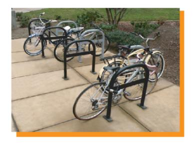
Properly installed inverted "U" racks allow for more bikes to be correctly secured in the same amount of space.
