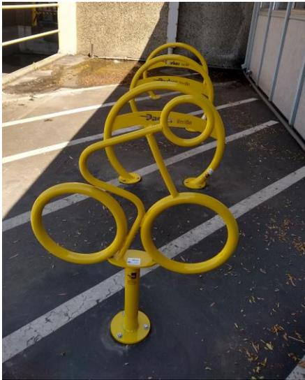
WCCTAC/511 Contra Costa staff worked with Parker Hannifin-Veriflo, in Point Richmond, to install three Omega style racks and one bicyclist style rack at their factory. The installation utilized asphalt anchors, which are new products that make installing in asphalt easier and cheaper, opening up more possibilities for bicycle rack locations.
