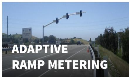
**Benefit:** By adjusting green times, adaptive ramp metering improves traffic flow onto I-80 and reduces merging collisions.
