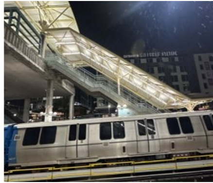
Figure 2: Millbrae Station AFTER LED Lighting Upgrade
