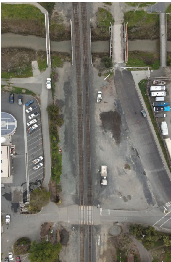
Drone footage of the project site and The San Francisco Bay Trail connection.
