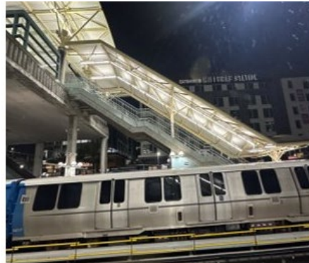
Figure 2: Millbrae Station AFTER LED Lighting Upgrade
