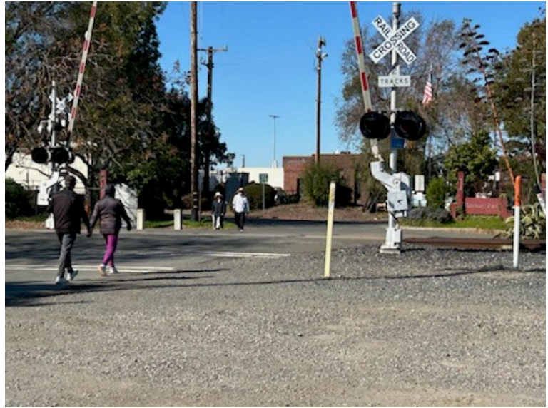
Existing at-grade railroad crossing with no designated safety zone for accommodating bicycle and pedestrian crossings.
