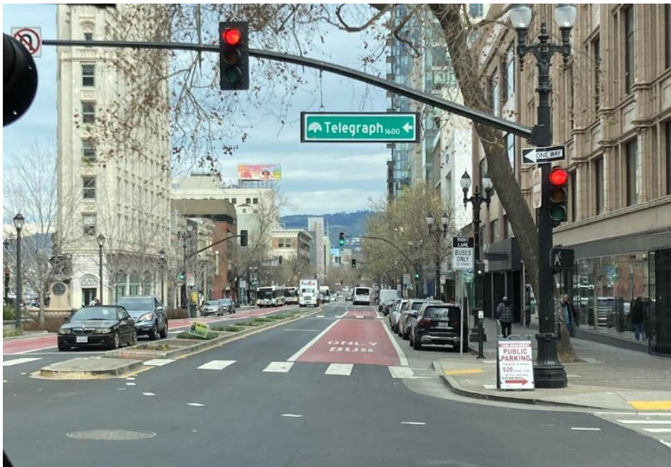
Side running with red painted bus lane and on-street parking
